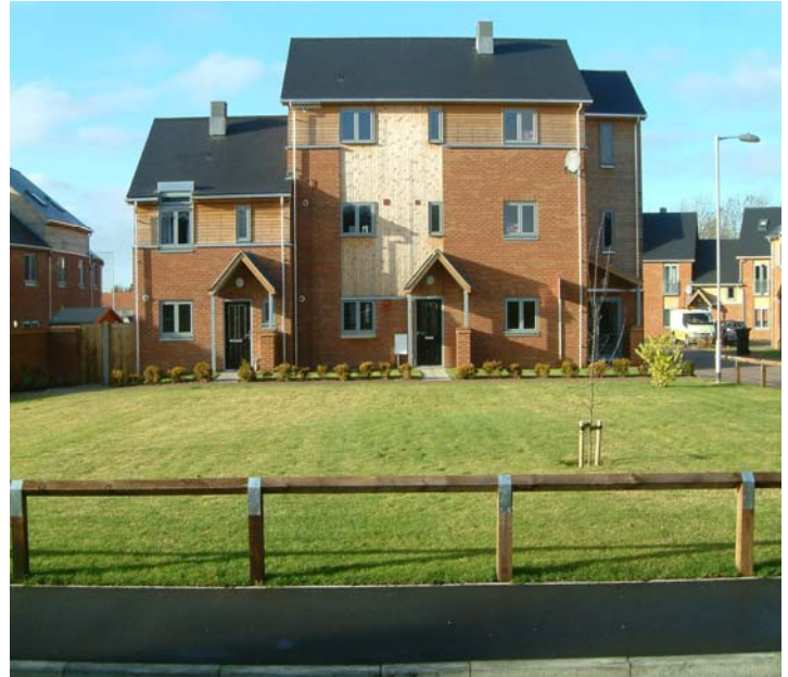
The development of 65 affordable homes by Broadland Housing, Norwich Road, Dereham.
