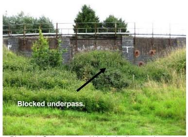
Picture 8: Overgrown and blocked railway underpass.
