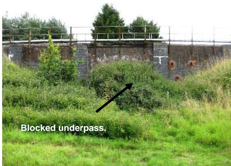
Picture 8: Overgrown and blocked railway underpass.
