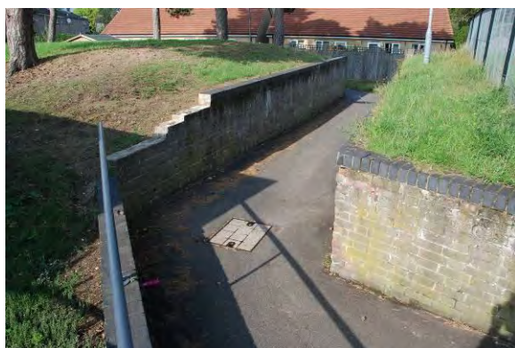
1.7m pinch point in 2.5m wide path. In the background is the first of two 45° bends – see right
