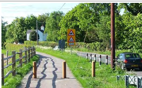
Row of bollards at 1.5m centres (Worth Way, West Sussex)
