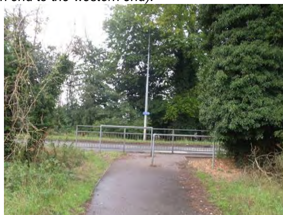
Staggered barriers to slow cyclists on approach to footway.
