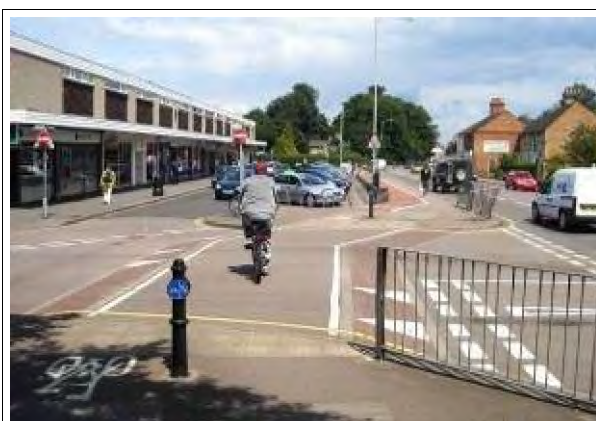
Example of an existing, good specification, ramped, priority crossing on a shared-use path (Bedford)
