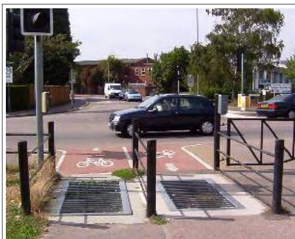
‘Cattle grid’ arrangement in central Cambridge permitting easy access to a path crossing an area grazed by animals. Simpler, ‘single lane’ designs would be applicable on the Thetford Loops.
