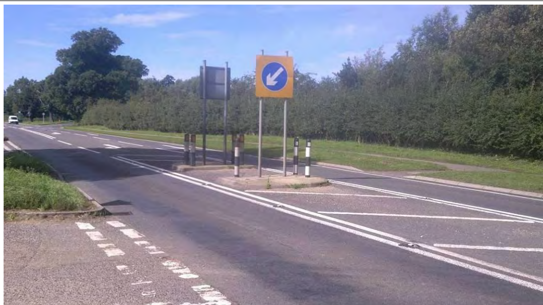
Protected refuge crossing on a 60mph Principal Road. A148 Sculthorpe, Norfolk.
