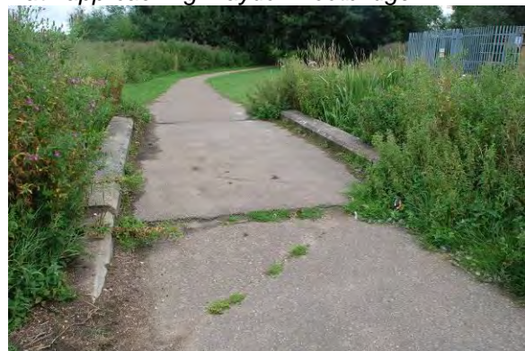
Bridge over tributary or drain showing poor surfacing
