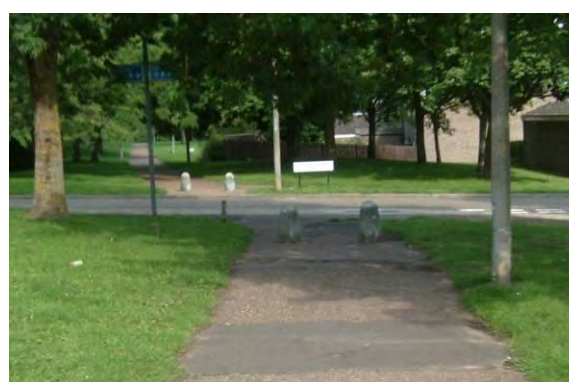
Facing east along footpath across Anne Bartholomew Road – note the absence of flush kerbs
