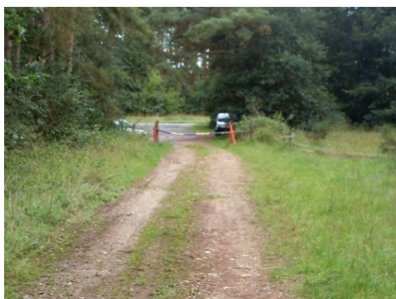
Gate to prevent vehicular access causes a barrier for cyclists.
