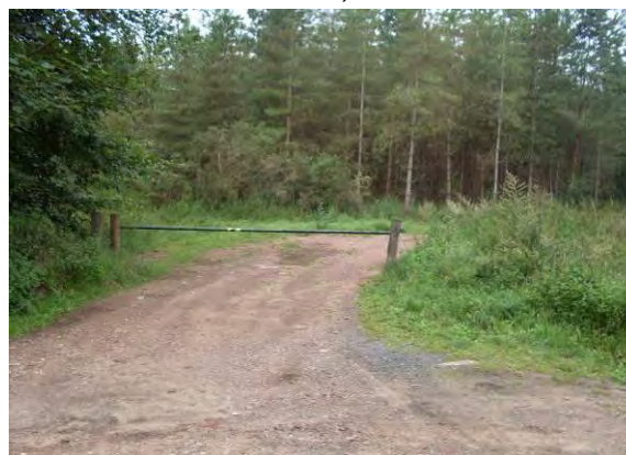
Gate to prevent vehicular access. Narrow gap provided for cyclists and pedestrians to pass.
