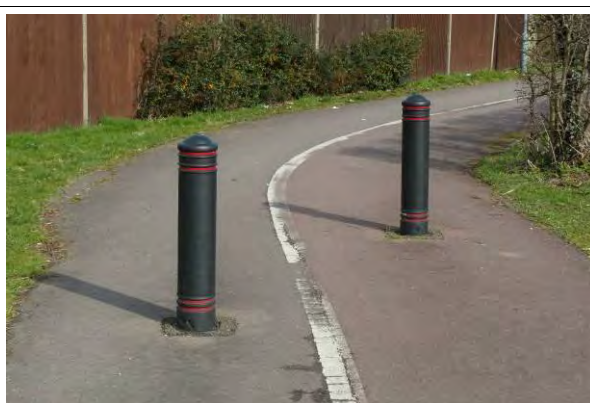
Staggered bollards to slow cyclists (Aylesbury)
