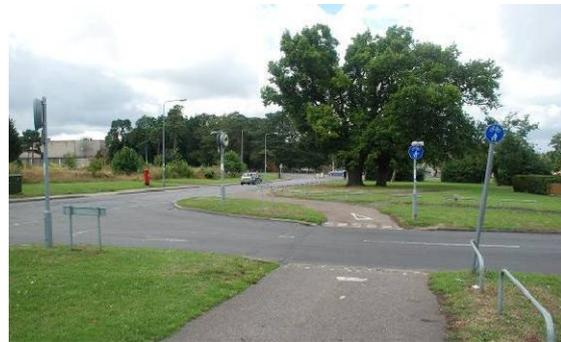
*Photo 13 – Existing crossing of Kimms Belt: a good example with flush kerbs and good sightlines*
