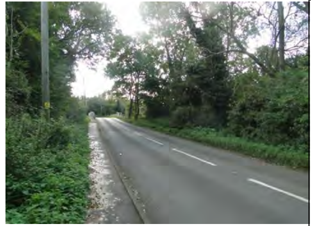
Looking south along Richmond Road towards the Parish boundary
