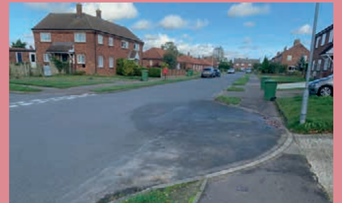
Excessive hardstanding and passing lay bys. Attleborough.
