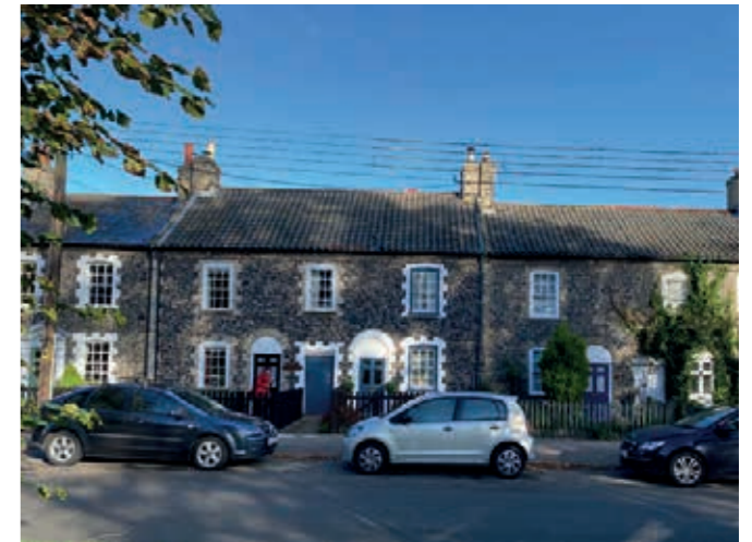
The Brecks - example of local urban vernacular architecture - simple double depth plan form, in knapped flint with gault dressings, with pantiles and slate roofs. Thetford.
