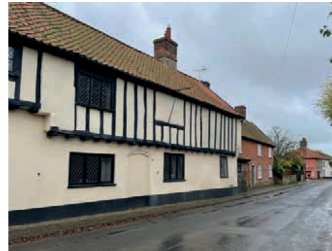
Higher status timber frame house with flint and brick base and jettied timber frame and close studs at first floor, pantiled roof. Bawdeswell.
