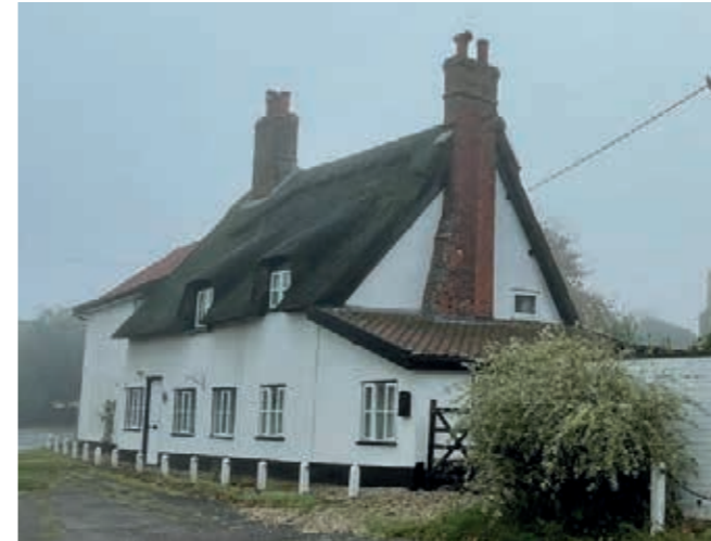
Timber framing with rendered clay lump infill, red brick chimney stack and thatched roof with pantiles to single storey extension. Great Ellingham.
