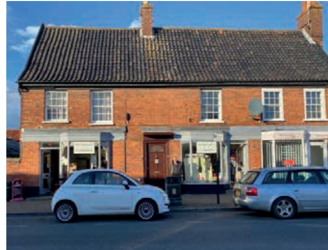
Red brick façade on clay lump and black pantiled roof. Watton.
