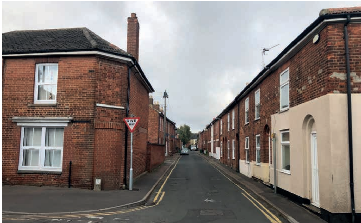
19th century terraced housing is a feature of areas around the town centre fringe, reflecting the town's growth in the industrial period
