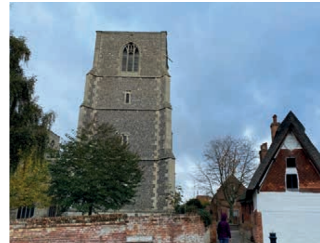
St Nicholas' Church is situated to the west of the town centre and is a key landmark.
