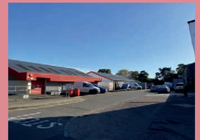
Extensive hardstanding and poor pavement provision. Thetford.
