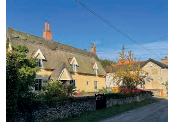
Timber frame with rendered and colourwashed wattle and daub and thatched roof with gabled dormers. Garboldisham.
