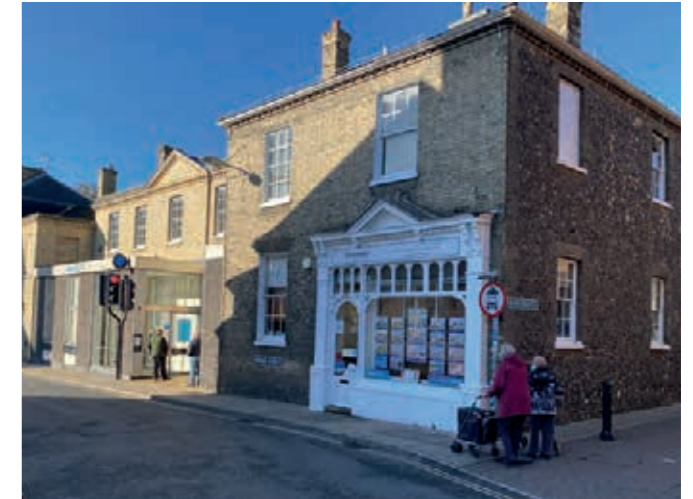
Gault brickwork with flint flank wall. Thetford.
