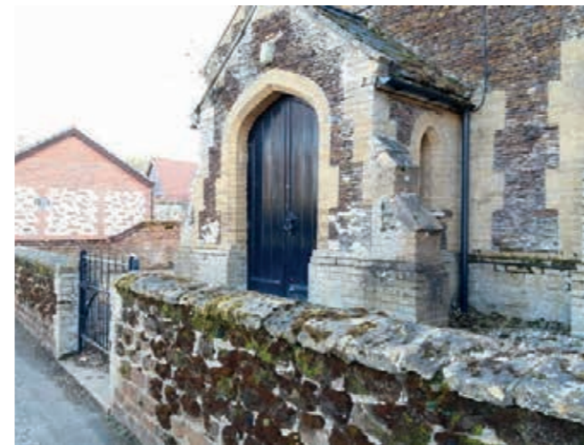
Carstone used on façade and boundary wall with gault dressings, Narborough with red brick and chalk wall in backdrop
