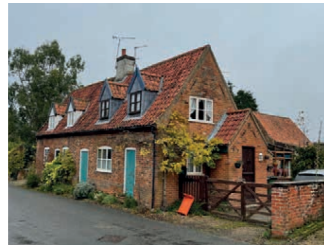
Single storey with attic cottages, built in red brick with chequer pattern, pantiled roof with gabled dormers. Mattishall.
