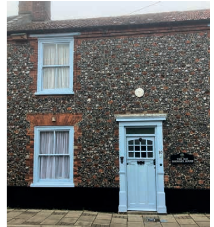
Knapped flint façade with red brickwork dressings and pantiled roof. Swaffham.
