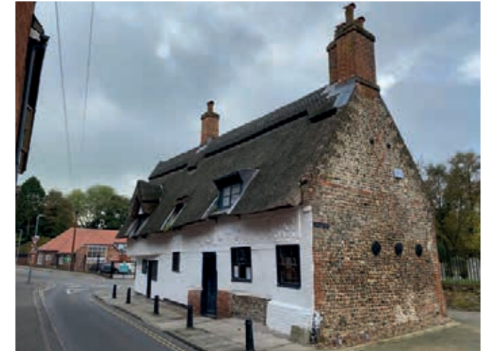
Single pile timber framed cottage with plastered façade and pargetting under eaves. Flint and red brick gable wall with red brick dressings and diapers and thatched roof. Dereham.
