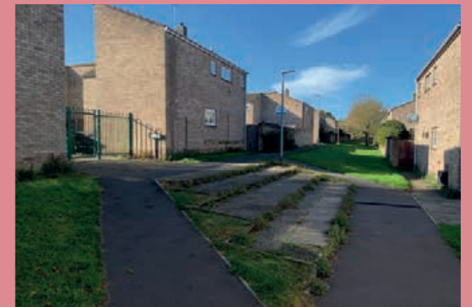
Poorly maintained public realm. Thetford.
