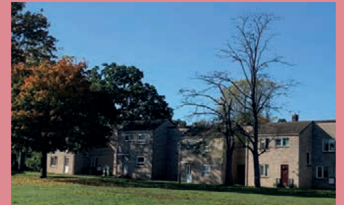
Buildings front attractive communal green space. Thetford.
