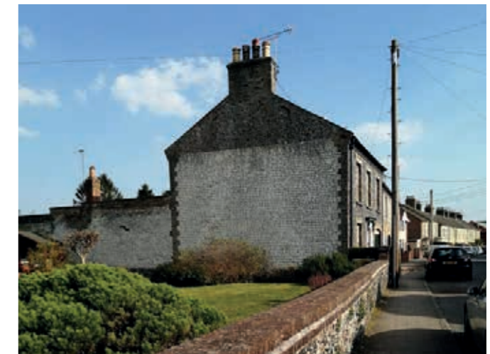
Chalk and flint on gable end, with knapped flint and gault brick façade and slate roof. Thetford.
