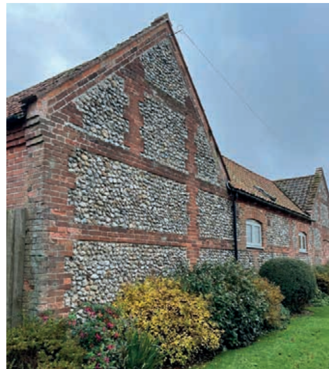
Rough flint with red brick dressings on converted agricultural buildings. Beeston.
