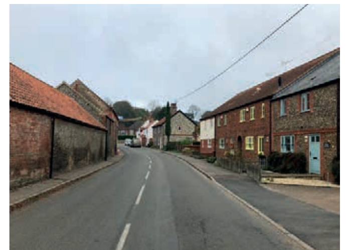
Mid-Norfolk - example village street scene with local vernacular materials and architecture - simple forms using flint and red brick, with pantiled and slate roofs. Litcham.
