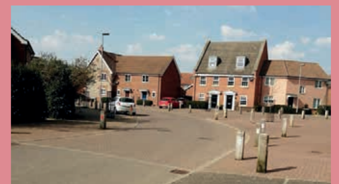
Large areas of hardstanding and bollards create a cluttered streetscape and lack soft landscaping elements. Dereham.
