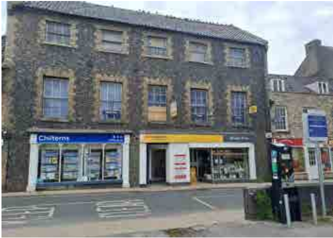
12-16 Bridge Street with rotten and blocked in sash windows giving the building a vacant appearance on the upper floors
