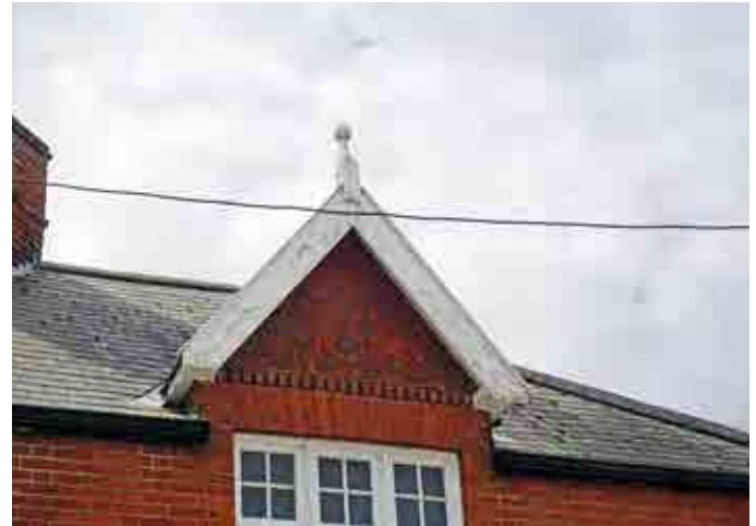
Flaking paintwork on the bargeboards of a building on Old Market Street
