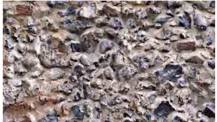
Inappropriate cement repointing of flint
