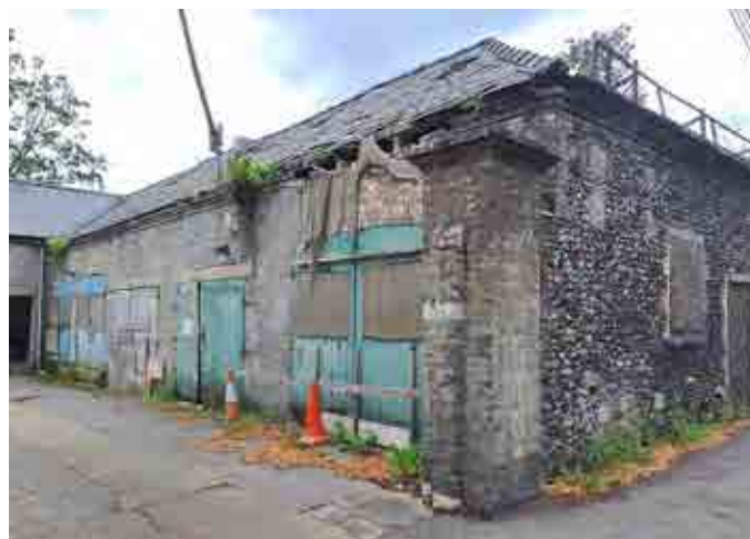
29a Bury Road with loose slates, vegetation growing within, missing brickwork and boarded up windows and doors
