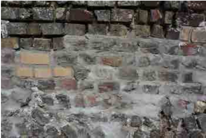
Poor repairs to brickwork including the insertion of inappropriate bricks
