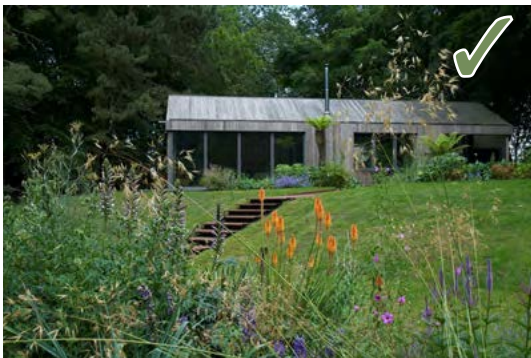
A simple building form is employed in this eco home, which reflects a traditional barn typology © Photo Ricard Hanson for Jeremy Stacey Architects
