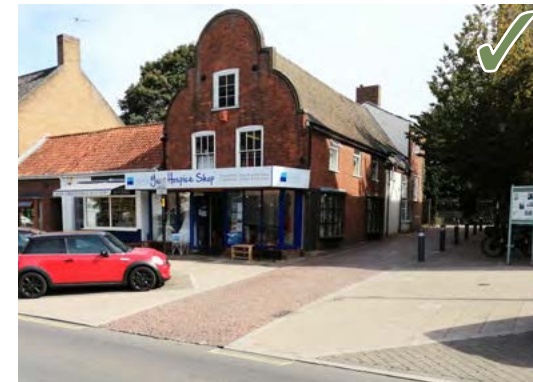
Materials and street surfaces can be used to mark different uses, users and street types, here demarcating parking spaces, pedestrian-only routes and shared surfaces in Swaffham. Non-standard materials need to be discussed with the highways authority, Norfolk County Council.
