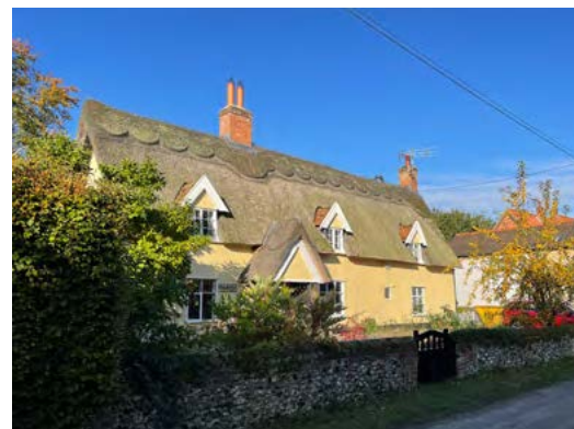
Timber frame with thatched roof, Garboldisham.
