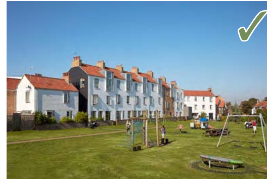
A terrace of taller buildings define and overlook an existing town green in Suffolk (© Ash Sakula).
