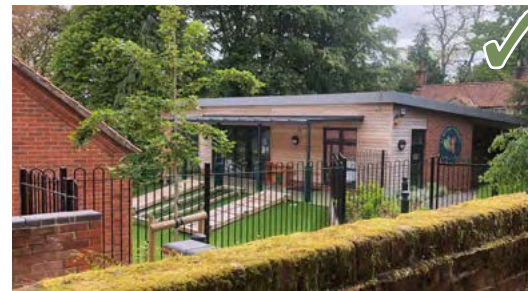
Contemporary primary school extension. Aylesham
