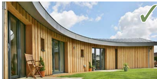
Passivhaus home in Swaffham, combining energy efficiency and low carbon timber cladding
