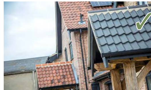
Well-designed materials and details add visual interest. The oak-framed porches add quality where people come into contact with it. Shipdham. © Clayland Estates
