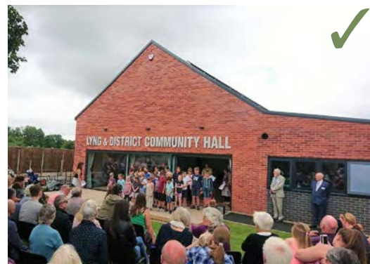
An atypical community building – a simple, well-detailed building form with good proportions and generous windows that look out onto a well-used garden area. Lyng Community Hall. © Photo Darren Leader for Charles Emberson Architect
