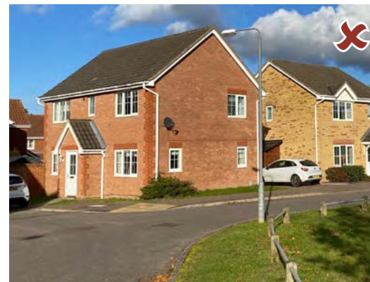
Small windows on the elevation facing this open space are not well proportioned. Buildings on a corner need careful design of all street facing elevations so they contribute positively to the streetscene and activate the street, and windows are a key element of this. Norwich
