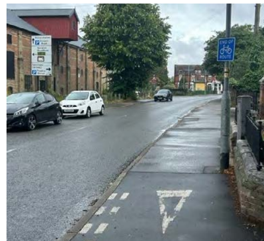
Poor example of cycle route transition to highway, Dereham.
