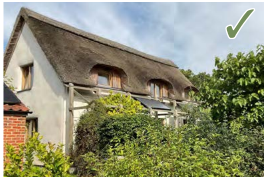
A simple building form that is a contemporary interpretation of a traditional timber frame house. Dormers add complexity but contribute to local character. This is an example of a Passivhaus. Hickling © Fran Bradshaw of Anne Thorne Architects
