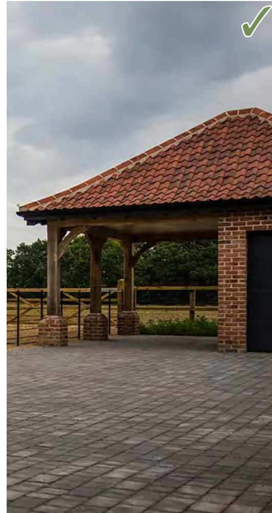
Reclaimed timber beams have been re-used as structural elements, Shipdham.
