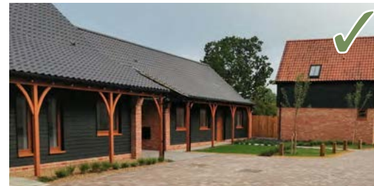
Bungalows are integrated into a building group in this development - The Gatherings, Great Hockham. © Ingleton Wood
