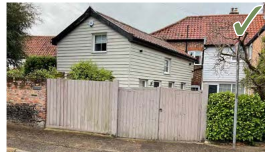
Contemporary extension in East Harling complements existing character by evolving rather than reflecting it.
