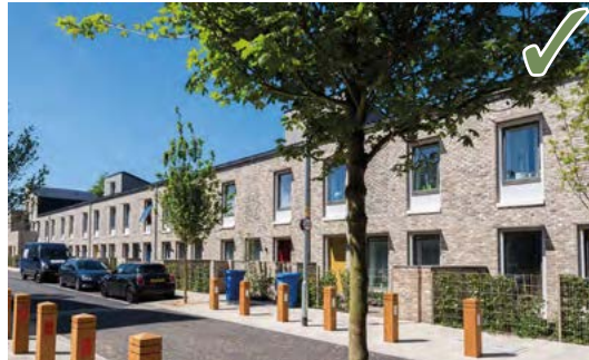
A contemporary interpretation of terraced housing. Goldsmith Street Norwich © Mikhail Riches & Cathy Hawley
