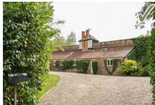
This house is bisected by a kitchen garden wall. It retains and integrates the wall's historic fabric into building that reflects the character of a traditional lean-to gardener's cottage, with a 'turret' that is a more contemporary interpretation. The Walled Garden, Garboldisham.
