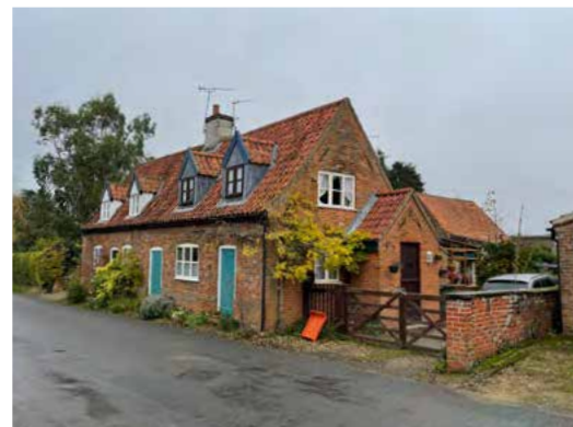
Red brick with pantiled roof, Mattishall.
