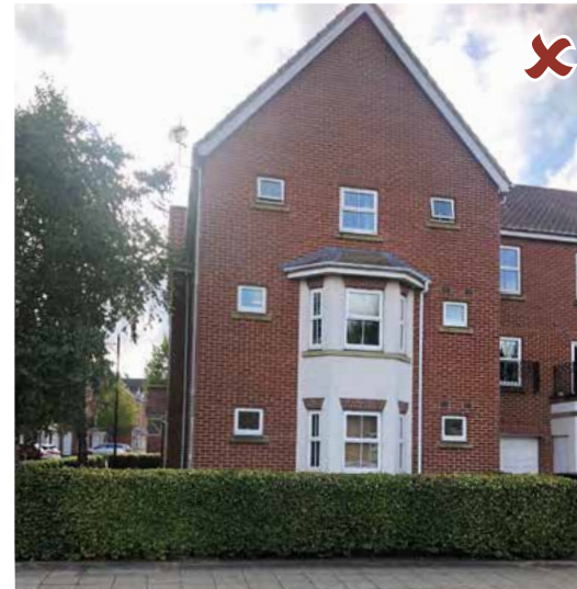
Small windows feel mean in relation to the size of the elevation.
