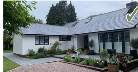
Photovoltaics integrated into a roof can reduce the visual contrast of its appearance (© GB-Sol).
