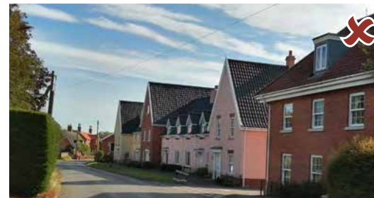
This street frontage is broken up by gables with steep roofs but their height and width makes them feel dominant and out-of-scale with the village street.
