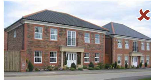
Large buildings set too close together, lacking any hierarchy of scale or proportions across the façade, standardised fake sash windows without reveals, or clumsy porch and roof details, all create a poor pastiche of historic character.
