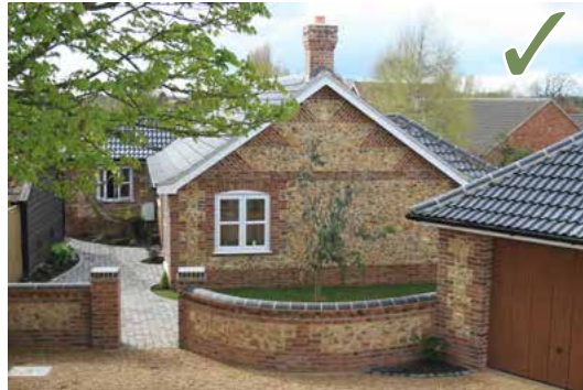
Texture, detailing, and materials have been used to create characterful façades in this example in Shipdham. © Clayland Estates
