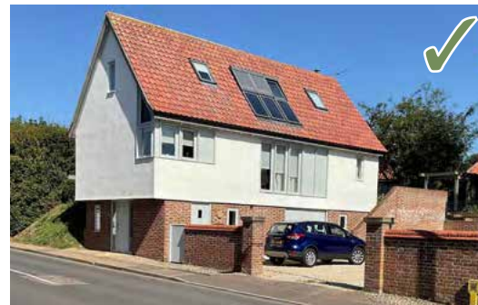
Contemporary interpretation of timber framed housing with simple compact form, articulated only by a jettied first floor. Wymondham © Lucas Hickman and Smith
