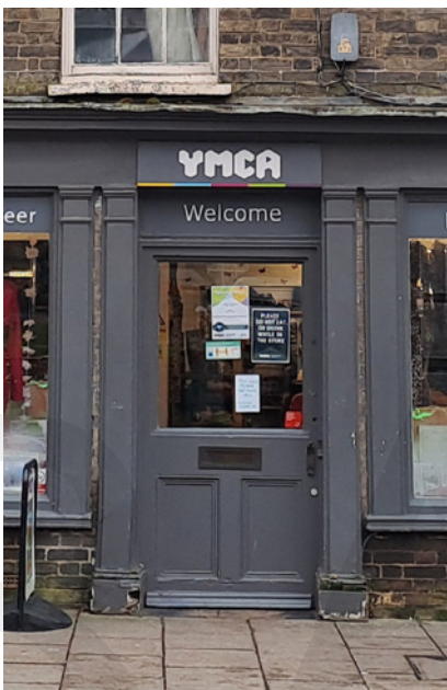
Replacement glazing within a historic timber shop door.
