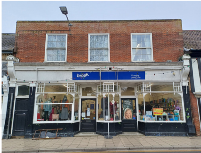
A Victorian shopfront with a high painted brick stallriser. Transoms divide up the shop window and horizontal divisions create top-lights. The stallriser and fascia are of a reasonable height, giving an overall balance and weight to the shopfront.
