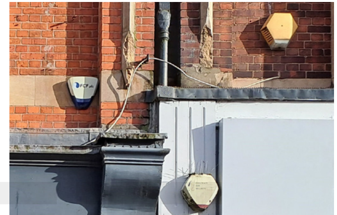
Redundant services, security alarms and wires create a cluttered appearance
