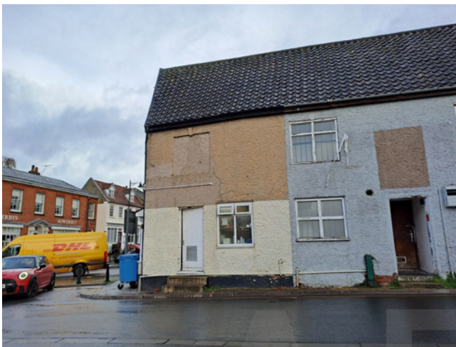
Buildings in poor condition on Quebec Street with cracked render and peeling paintwork to timber windows
