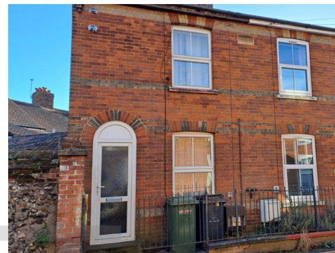
Inappropriate uPVC windows and doors eroding the historic character of both houses
