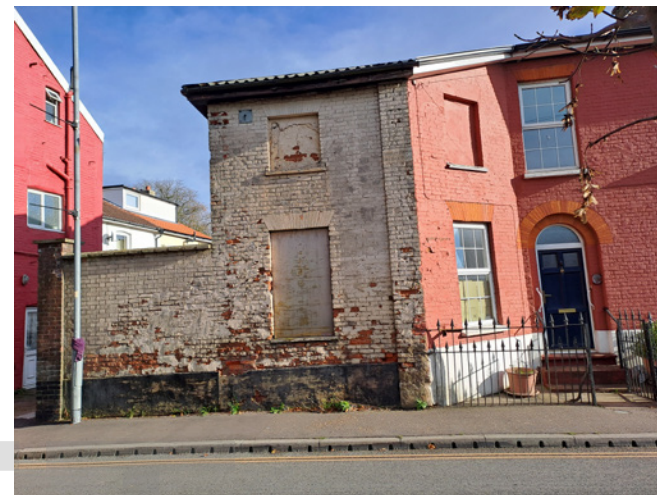
Flaking paint and crumbling brickwork on apparently vacant house on Commercial Road
