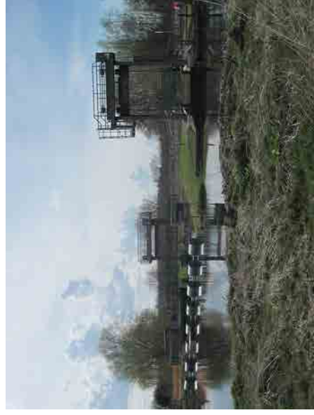
Brandon Lock & Weir limits the length of craft to 39' which are able to pass upstream to Brandon.
