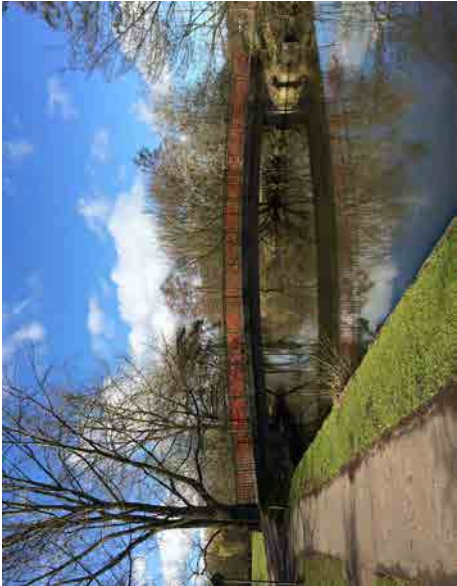
Blaydon Footbridge will need to be raised if the river is restored to full navigation.
