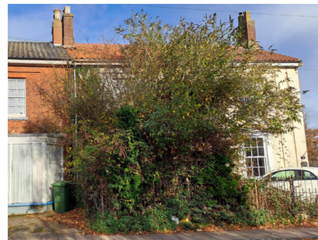
52 Norwich Street with an overgrown garden and railings and building façade behind in poor repair
