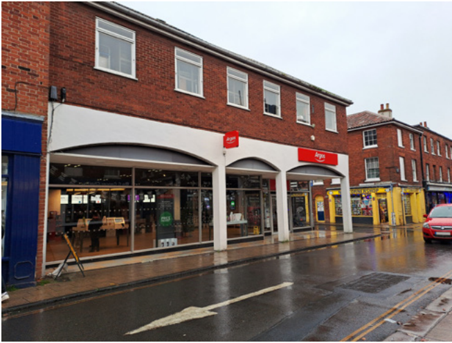
Long façade across several historic building plots with ground and first floor out of scale to neighbouring property heights.
