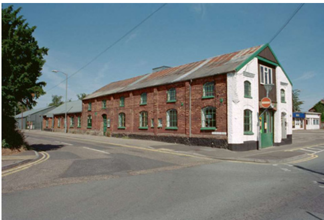
St Nicholas Works on Cowper Road, formerly W J Gidney's ironworks. (Dereham Heritage Trust)
