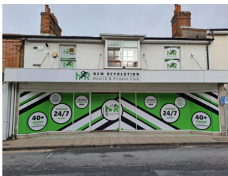
Overly large signage, too wide fascia and boarding blocking view in inappropriate for historic building above
