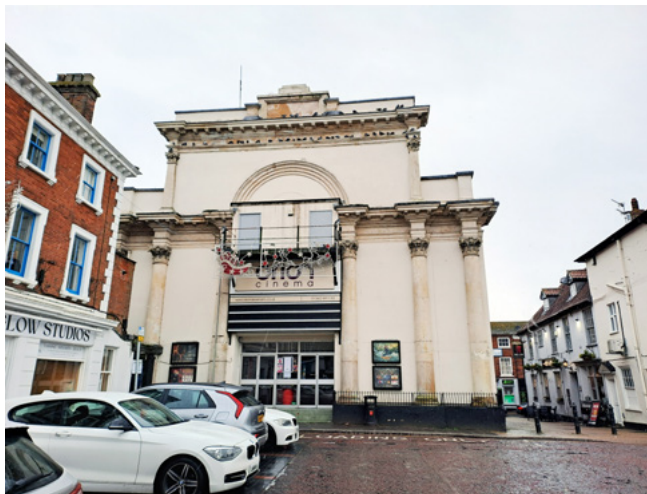
The former Corn Hall
