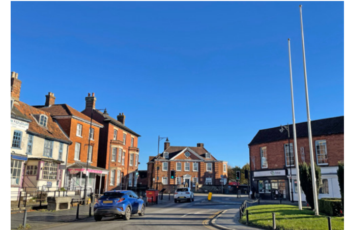
C View of Hill House from across the Market Place.
