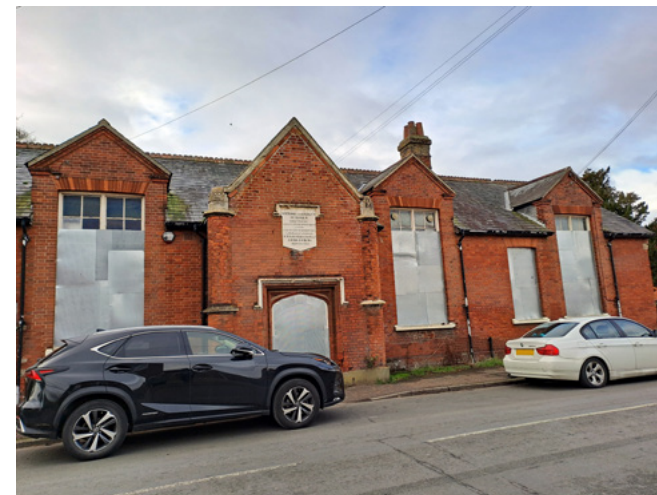
London Road School with windows boarded up due to vacancy
