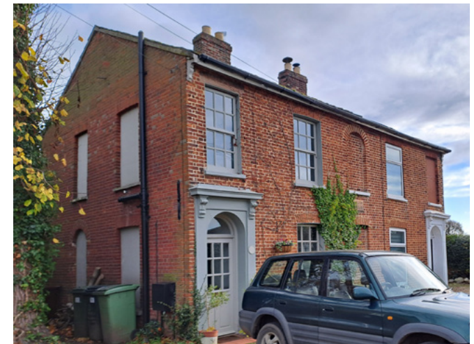
Attractive late nineteenth century semi-detached house with decorative corbelled door surround
