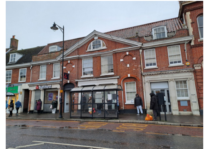
Modern bus shelter out of character with historic street and blocking views of historic shopfronts
