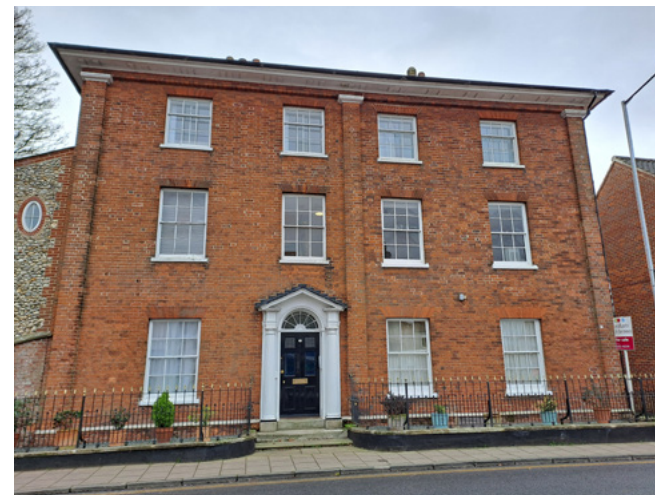
Example of a generally well-maintained building at the south end of High Street with timber sash windows and doorcase in good condition as well as repointing and painted railings.
