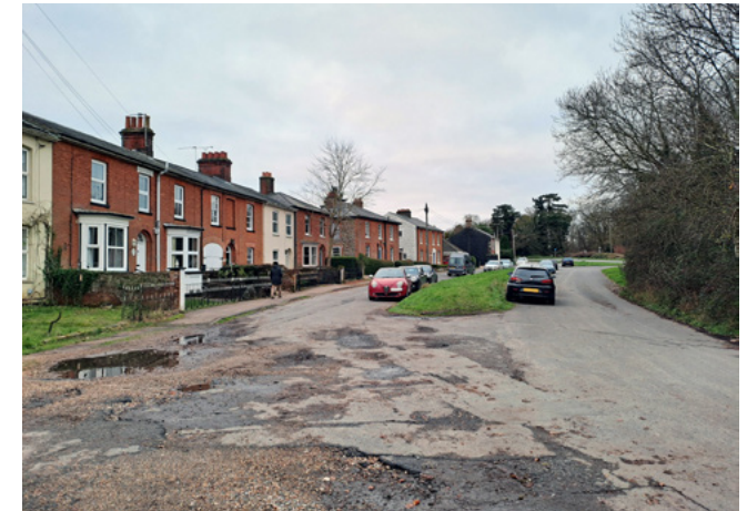
Patchy Surfacing along Dereham Road
