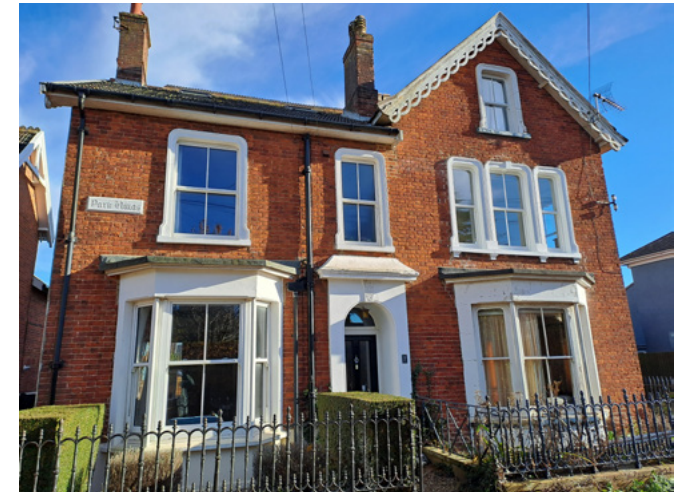
Larger Victorian villa on Park Road with ornate railings
