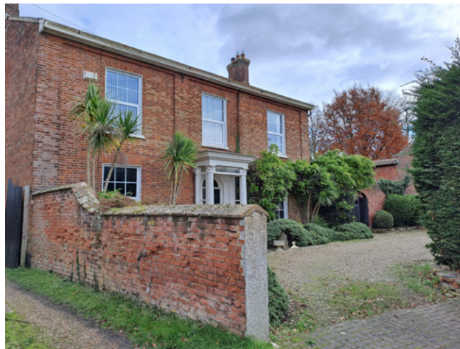
Attractive late nineteenth century villa
