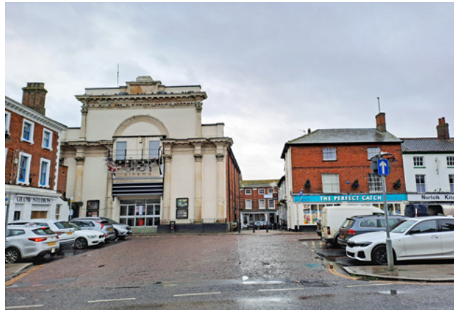
E View of the cinema (former Corn Hall) across the Market Place.
