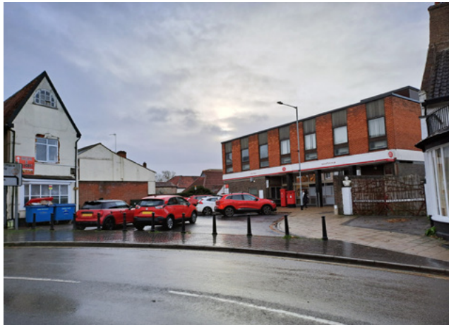
Hard landscaping around the Post Office unattractive and cluttered
