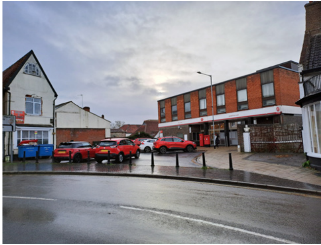
Post Office is out of scale with the surrounding buildings in height and width with a horizontal emphasis and materials such as wood panelling which does not characterise the conservation area.
