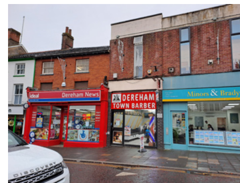
Large fascia obscuring historic shopfront on the right, garish signage and signage in windows clutters the street scene
