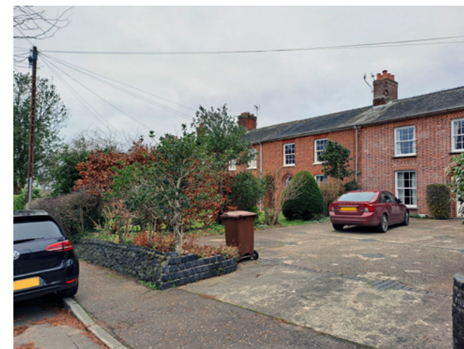
Terrace house with large area of hardstanding on Elvin Road not in keeping with historic character of the road
