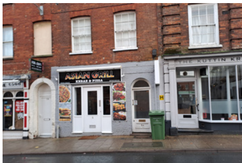
Historic shopfront window replaced with modern door and overly large signage inappropriate
