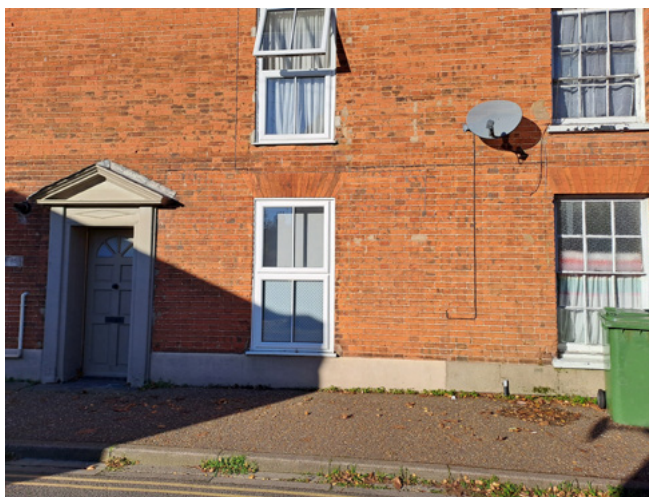
Inappropriate uPVC windows on a historic building, appropriate timber windows, though in poor repair, visible on the right hand building
