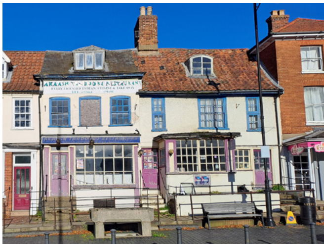
Vacant shop on Marketplace in a generally poor state of repair
