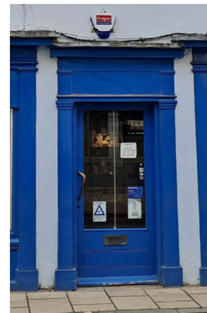
Historic shop doorcase containing door with large glazed panels.
