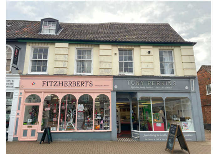
A traditional Victorian shopfront with large plate glass and delicate arches over delicate cast iron column transom divisions on the left. The stallrisers is in proportion with the shopfront.
