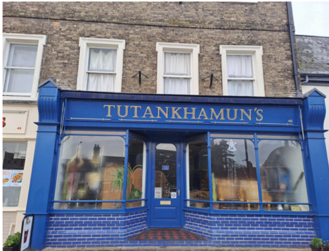
Traditional shopfront with a glazed brick stallriser and transoms and horizontal divisions breaking up the expanse of plate glass.
