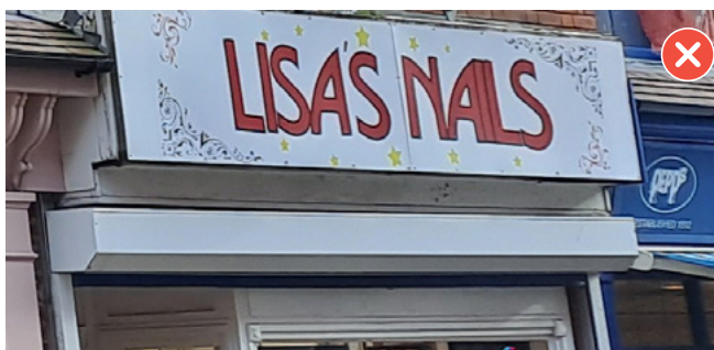
Example of a negative protruding box canopy
