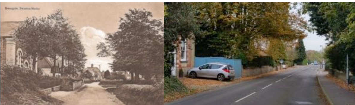
2.3.10. Greengate c. 1920 and recent view.
