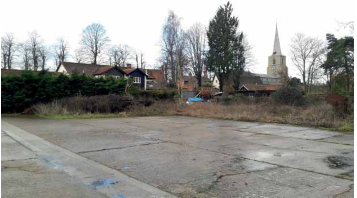
Plate 8 view south-west showing concrete yard surface within LP 003
