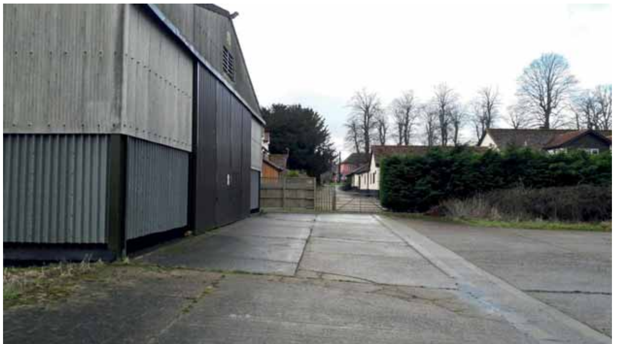
Plate 9 view south. The only clear view through to Church Green and the historic core of the village. Church Farm Barns of recent construction largely blocks the view. It became clear that at least from ground level many of the views were obstructed by new-build buildings and thick foliage. A view along the access road to Church Farm Barns gave a very obscured view back towards the PDS.
