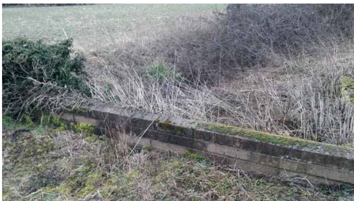
Plate 7 recent/modern bridge construction within LP 003
