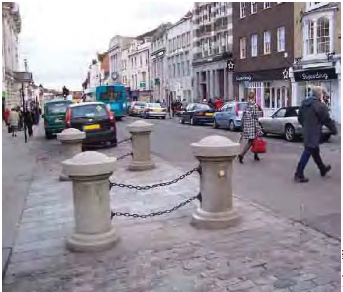
Figure 6.2 Informal crossing, Colchester – although the chains and a lack of tactile paving are hazardous to blind or partially-sighted people.
