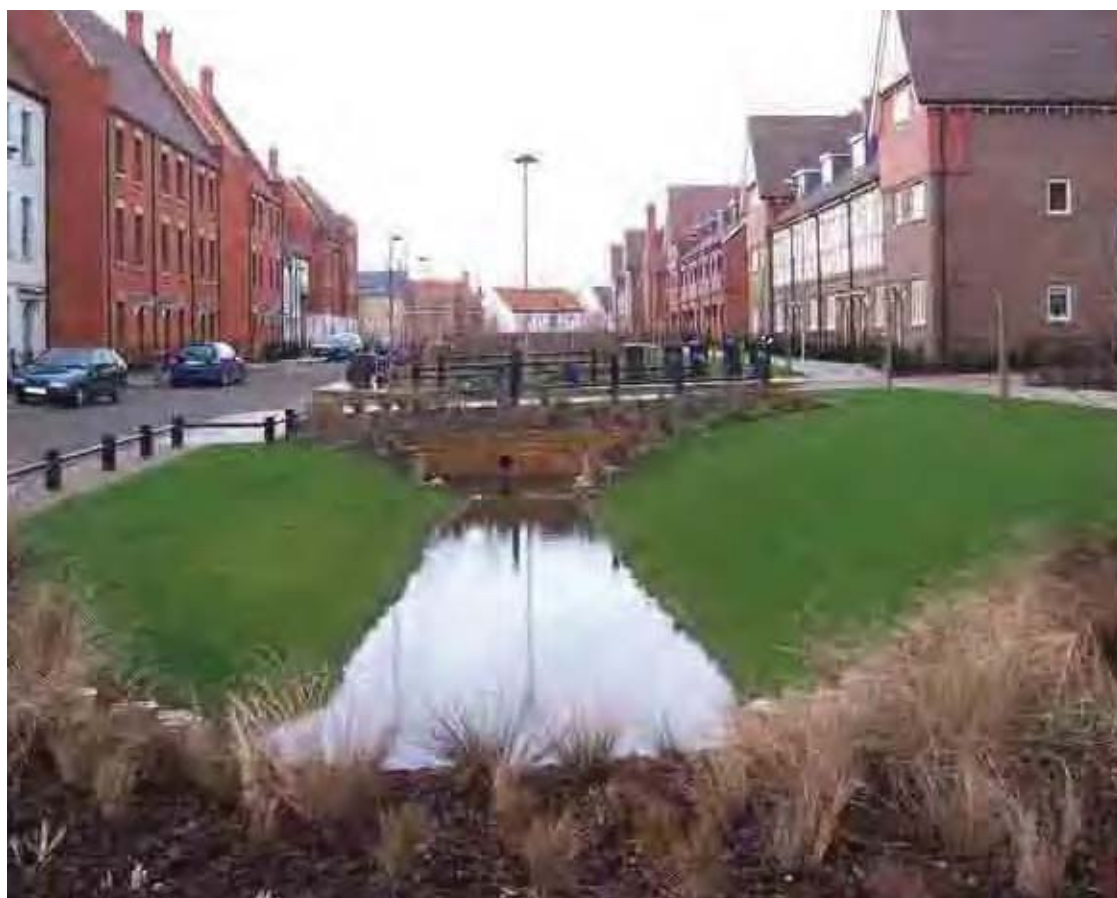
Figure 11.5 Sustainable drainage systems can form an integral and attractive part of the street.
