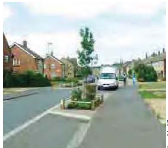
Figure 9.4 Kerb build-out defines parking area and provides room for planting clear of the footway.
