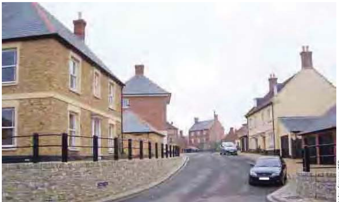
Figure 6.11 In some instances it may be possible to keep footways level when the carriageway is on a gradient, although this example deflects pedestrians wanting to cross the side road significantly from their desire lines.
