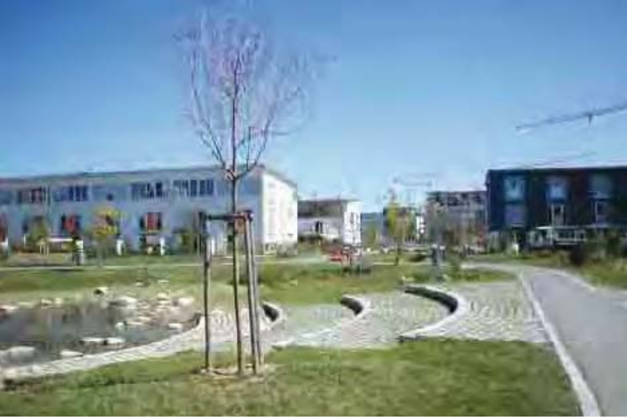
Figure 2.4 An example of a sustainable drainage system.
