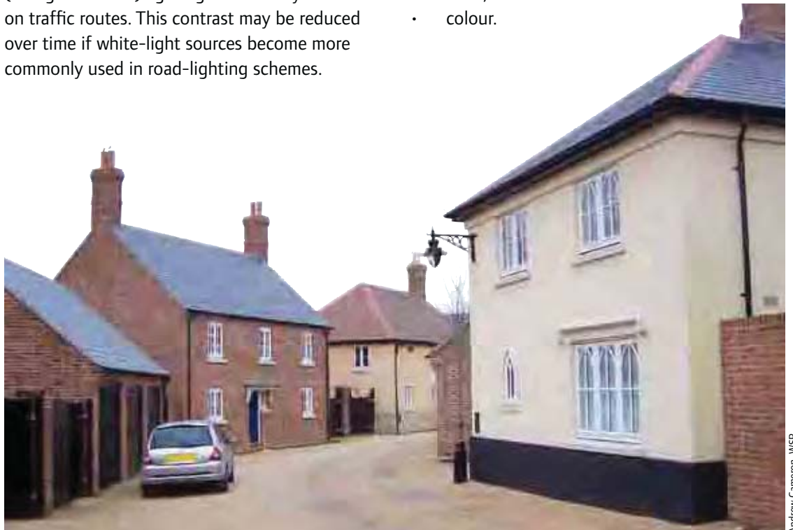
Figure 10.3 Street light mounted on a building.
