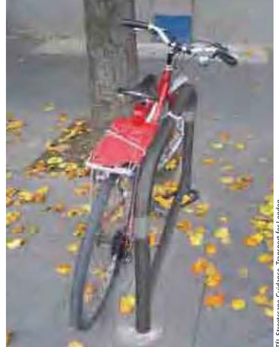
Figure 8.3 Sheffield stands are simple and effective. The design allows the bicycle frame and wheels to be easily locked to the stand. Note the tapping rail near ground level and the reflective bands on the uprights.
